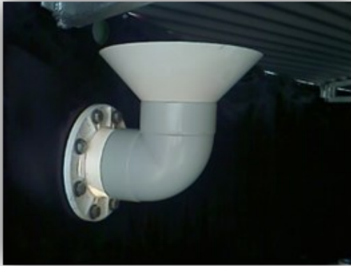
Internal view of our 150mm Bellmouth Overflow
